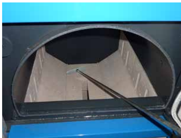
Sweeping the ash through the nozzle down into the bottom (cleaning) chamber. The opening in the nozzle must be always clean and free.
