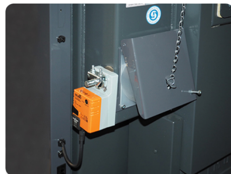
Belimo actuator and air damper
