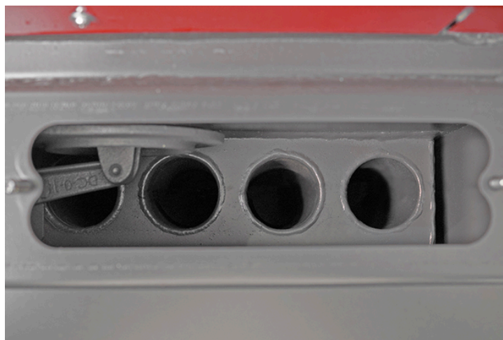
Tubesheets without air brakers
